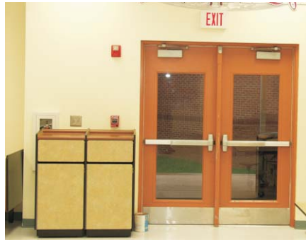
Trash receptacles placed near the exit door.
