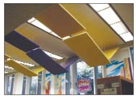
Pictured here are 2" thick sound baffles hanging in a cloud formation to help keep the noise down while creating a bright exciting area for your dining room.
